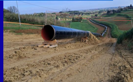
Adriatic Line construction
